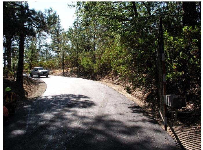
High Valley Road after resurfacing.
