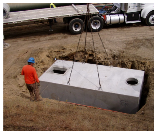
Installation of rainwater collection tank
