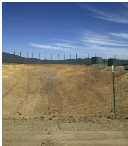
West Coleman Sump floor and wall
